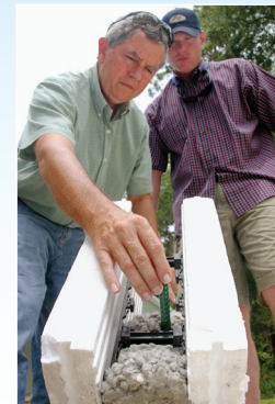
Extension activities encourage the use of energy-efficient, wind-resistant construction materials such as insulating concrete forms (ICFs).
